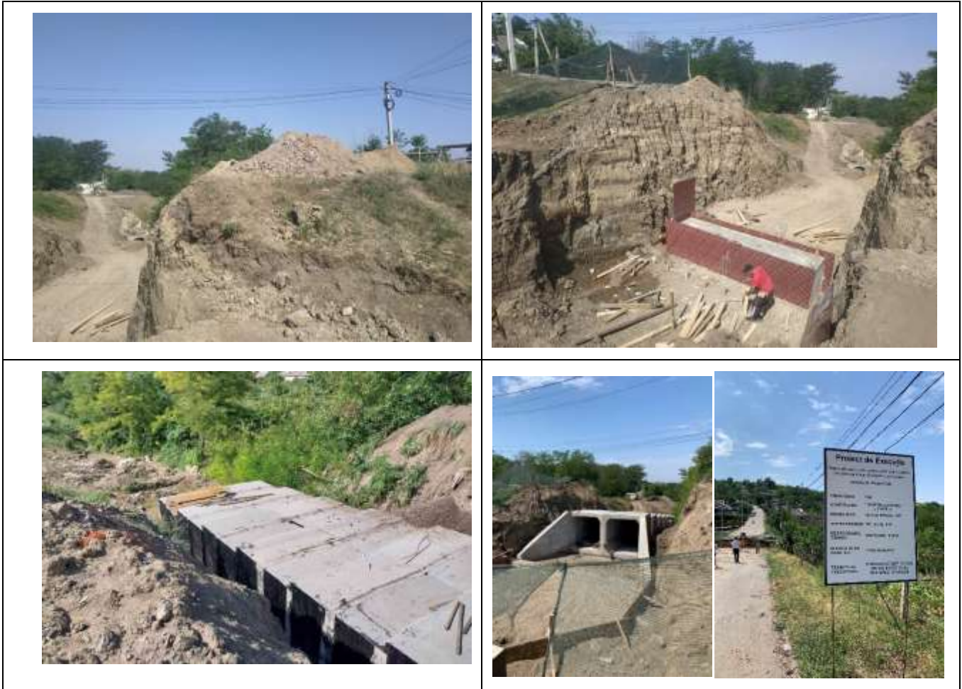
Construction process of Causeni road
