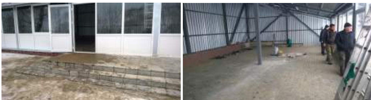
Fig. 13. Construction of agricultural market in Sarata Veche village, Falesti district
