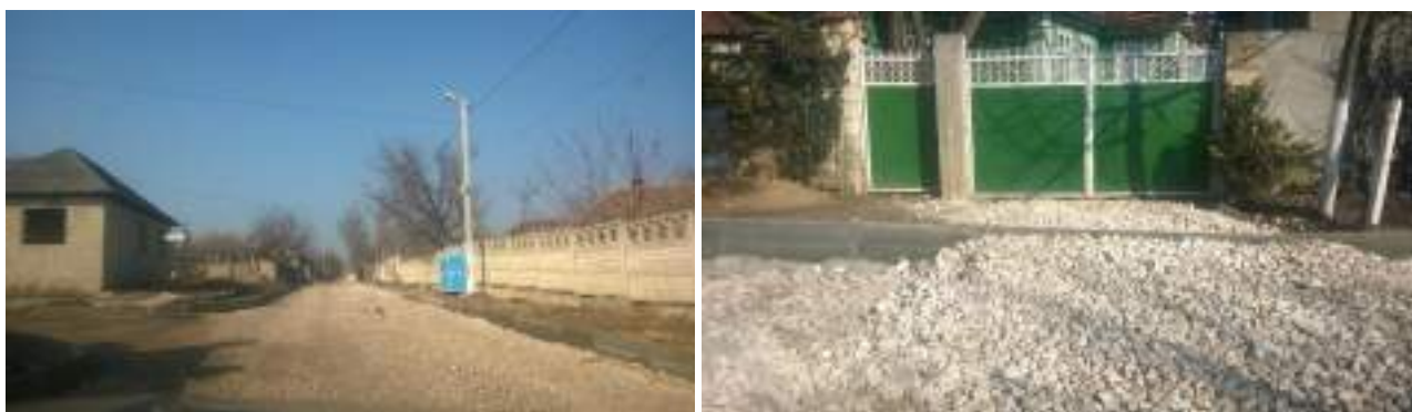
Fig. 14. Civil works of compacted concrete road segment with a length of 0.86 km
