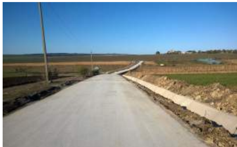
Fig. 11. Civil works for construction of concrete road with a length of 2,04 km in Hiropul Mare village, Criuleni district
