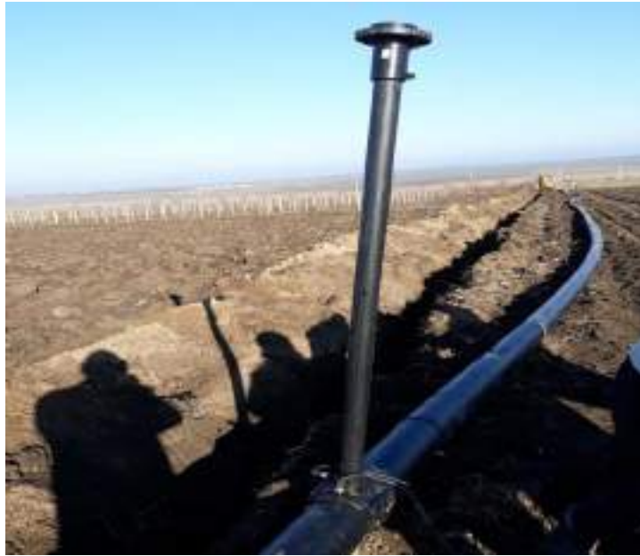
Fig. 7. Civil works for construction of water supply network for irrigation with a length of 3,762 m in Telita village, district Anenii Noi.
