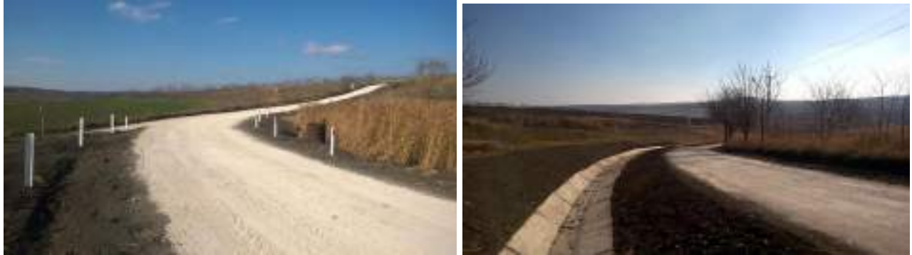
Fig.12. Construction of a white variant road segment with a length of 1,8 km in Bilicenii Vechi village, Singerei district
