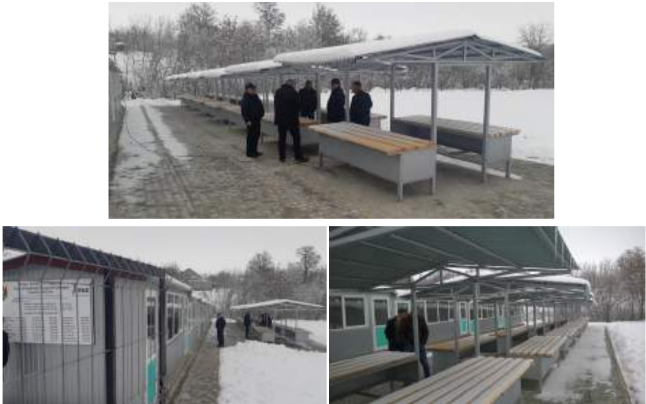
Fig.10. Civil works for construction of agricultural market in Mihaileni village, Riscani district
