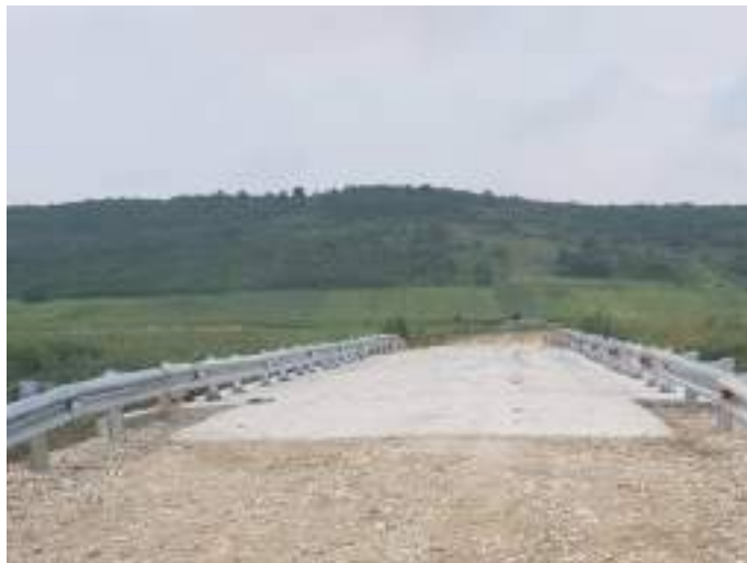
Fig.8. Civil works for bridge construction with access over Cogilnic river towards production zones in Stolniceni village, district of Hîncești.
