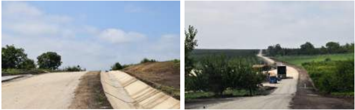
Fig.9. Civil works for construction of white variant road segment with a length of 1,67 km in Saghineni, Alexeevca village district of Ungheni.
