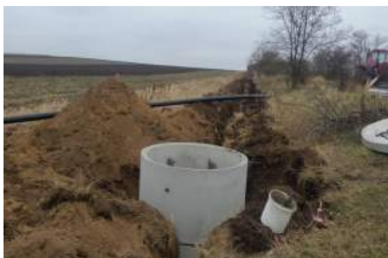
Fig. 6. Civil works for construction of water supply network for irrigation with a length of 3,762 m in Telita village, district Anenii Noi.
